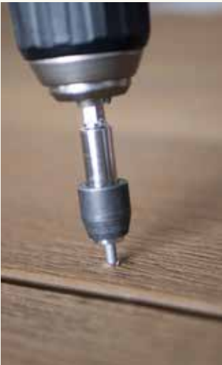
Screw driven below surface with drill; Lastane layer begins to compress around the fixing.
