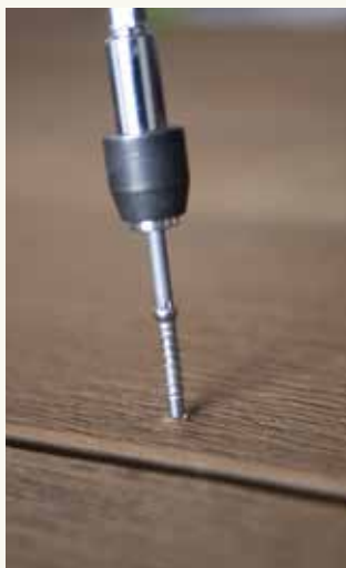
Screw aligned above board surface prior to installation using Durafix® screw and driver bit.
