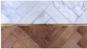
**Design requirements:** The tile bar is attached directly to the tile (not the wooden plank) and must be installed by the tiler prior to the wood floor being laid. When installing the timber, it should finish 2-3mm from the tile bar (to allow for expansion).
