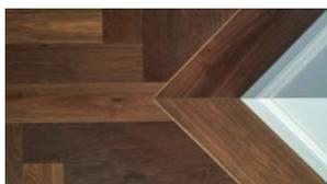
**Design requirements:** The bar should be fixed to the transition edge with screws with the top of bar set level with the top of the flooring.
