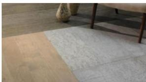
**Design requirements:** Experienced installers can make a ramp from the product being installed for a perfect colour match. Where possible, ramp down in an inconspicuous place like a doorway.
