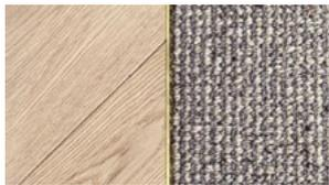
**Design requirements:** The top of the flat bar should be set level with the top of flooring.
