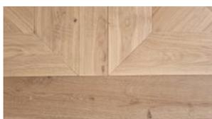
**Design requirements:** If you are not planning to use an extruded flat bar when adding a border or creating a break in your flooring, then where possible a T&G profile should be used to join the boards together. Sometimes this is not possible (where the profile has been removed).
